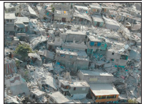
TOP: Vadim Levtonyuk (standing to the left, wearing an orange shirt, dark vest, and pants) and his companions wait to leave Port-au-Prince airport. BOTTOM: Dozens of the thousands of buildings that collapsed in Port-au-Prince. Photos courtesy of Slavic Full Gospel School.
